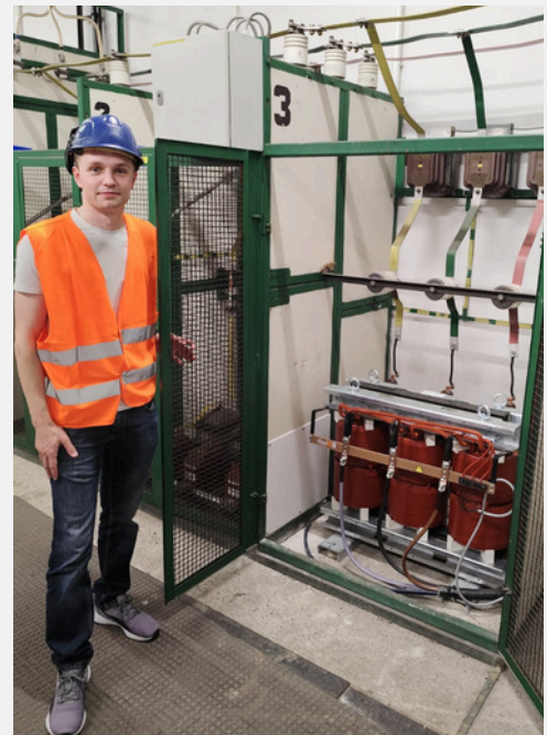
Photo: Andrzej Seget Junior Key Account Manager Elhand Transformatory. Product: ET3H o mocy 74kVA i napięciach 6300V//145V
